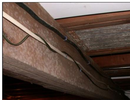
*Aspergillus mold on joist and subfloor*
