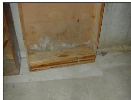
*Mold on set of shelves; note efflorescence at bottom of foundation wall*
