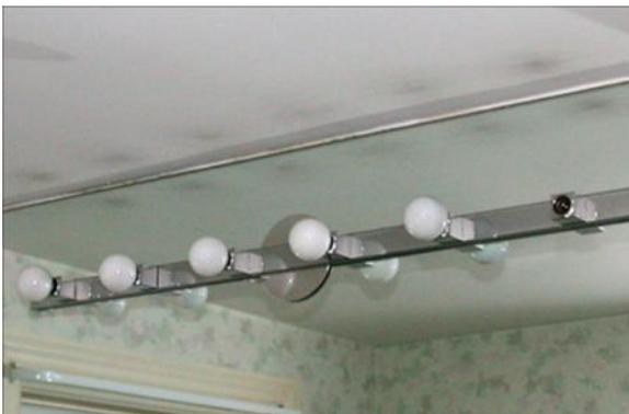
*Soot stains above bathroom lights due to jar candles; such staining can also be due to soot from spillage of combustion products from an oil burner.*
