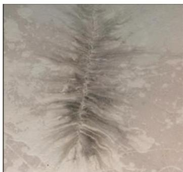
*Air flow through a floor crack carried smoke and soot across ceiling cavities from a fire in a distant condo unit*
