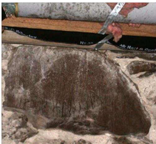
*Condensation of moisture on a cool crawl-space foundation wall: vapor to liquid. Mold is growing on the flexible duct due to high relative humidity.*
