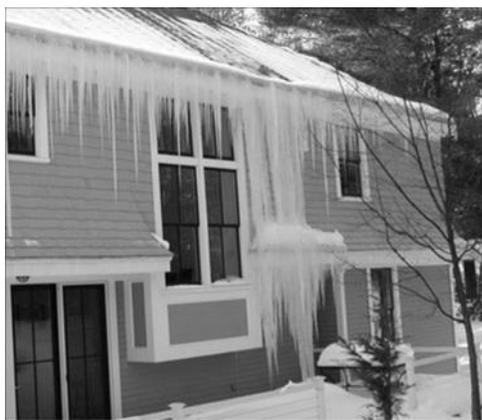
*Ice damming: Liquid to Solid. The large icicle destroyed the deck when it fell.*
