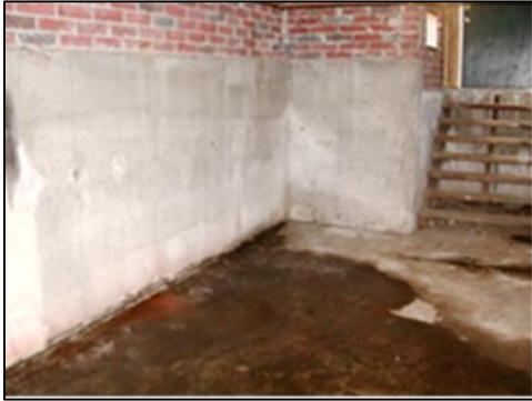
*Basement water near the bulkhead*
