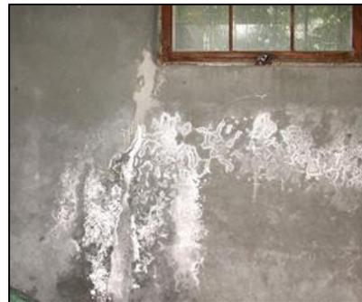
*Efflorescence on a foundation wall*
