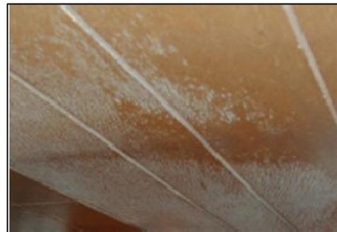
*Mold growth on a paneled basement ceiling*
