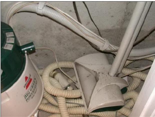
*Mold-growth spots on a foundation wall and vacuum*
