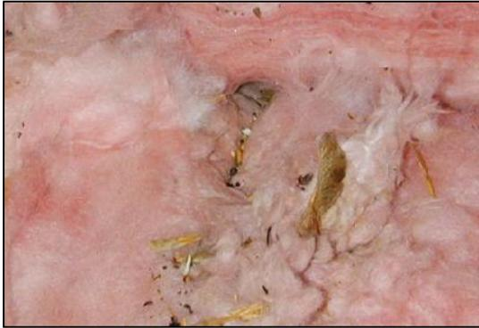
*Mouse burrows and droppings in fiberglass insulation*
