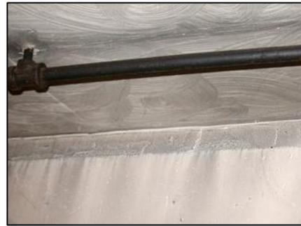
*Soot streaks on foundation wall and ceiling from oil burner spillage*
