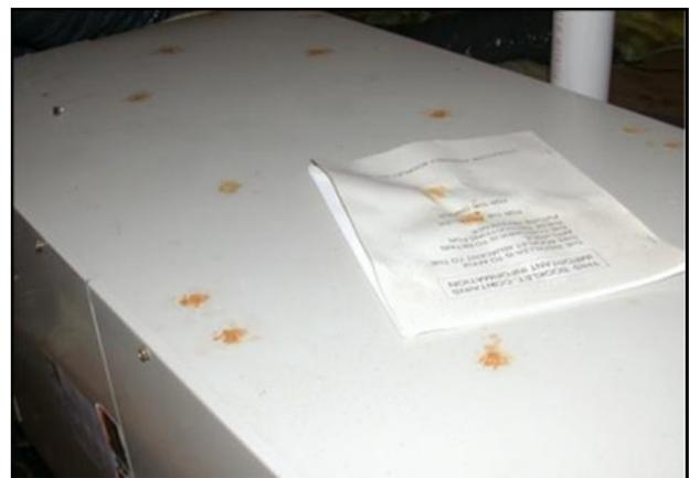
*Rust stains on attic AHU from nail drips*
