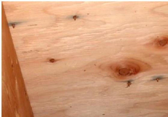
*Black stains at nails from condensation are not mold*
