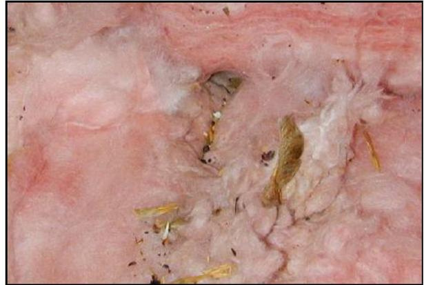
*Mouse burrow and droppings in attic insulation*
