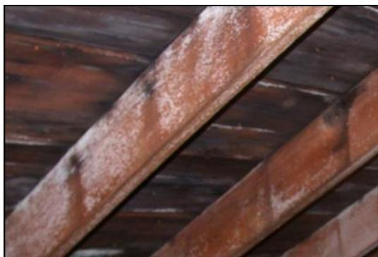
*Truss mold inhibited by zinc run-off from nails*
