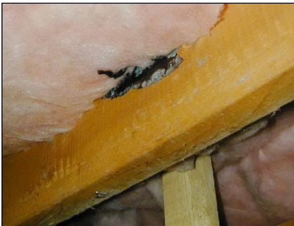
*Mold growth on rodent urine on ceiling joist*
