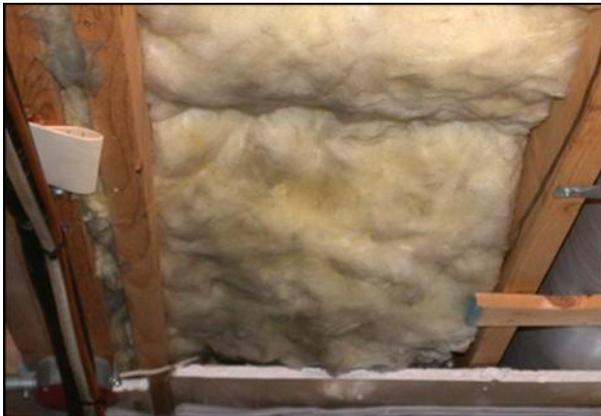
*Soot from combustion spillage looking like mold*
