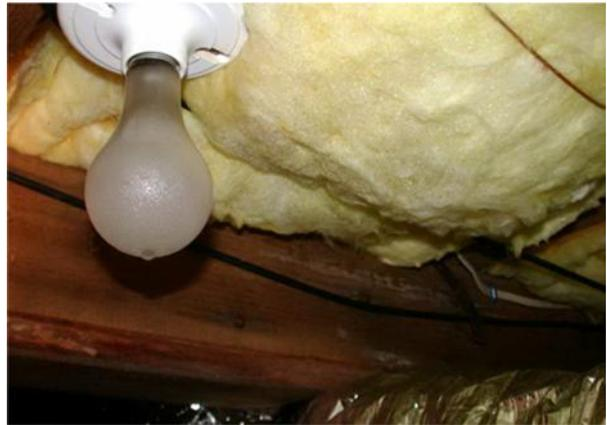
*Condensation on a basement lightbulb and on fiberglass insulation [note the rusty insulation support]*
