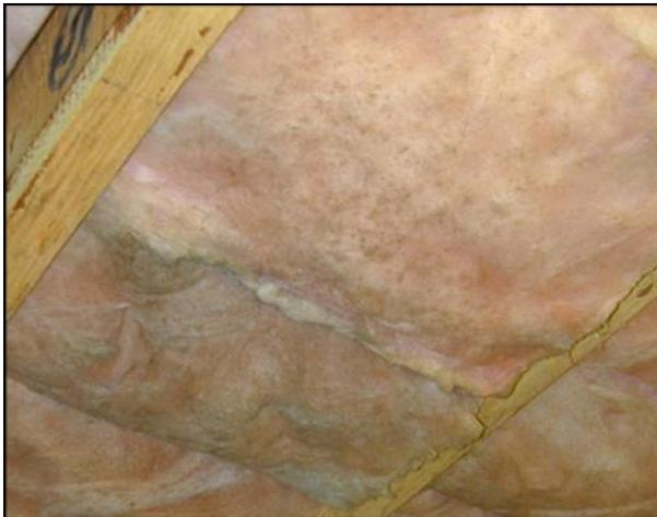
*Visible mold spots [a rarity!] on fiberglass ceiling insulation*
