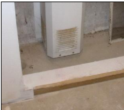
Mold growing in dust on Humidex intake
