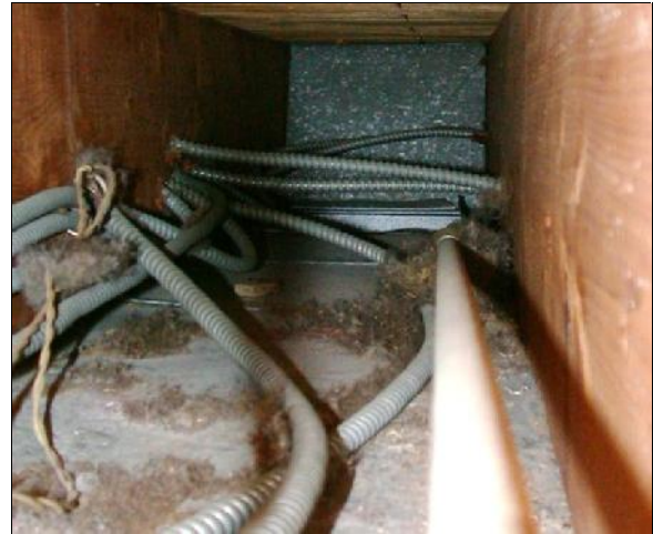
How can this panned bay ever be cleaned? May Indoor Air Investigations LLC
