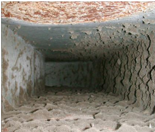
A soiled return; airflows created the pattern May Indoor Air Investigations LLC
