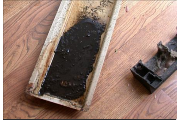
Refrigerator drip tray soiled with microbial growth May Indoor Air Investigations LLC
